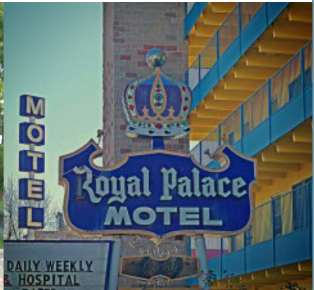
The largest parcel without a tenant at 46,000 sq. ft. This former hotel sits vacant
